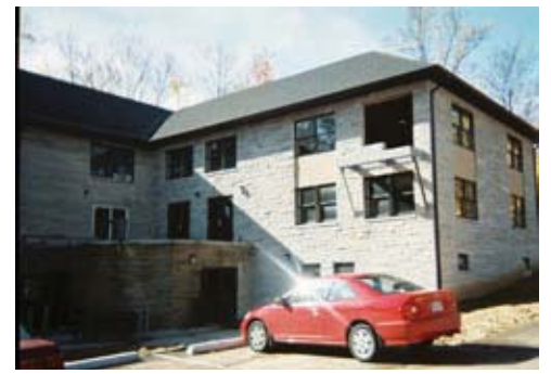
Back courtyard, showing part of the expanded, paved parking lot, the elevated patio, and new ground floor.
